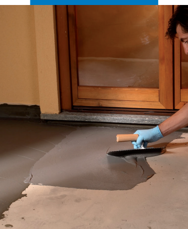
Waterproofing of terraces by trowel
