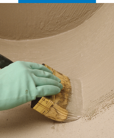
Waterproofing of details by brush
