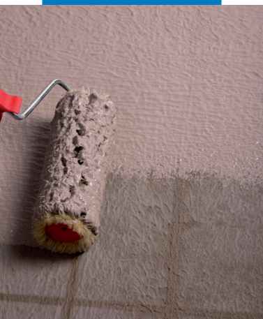
Waterproofing of details by roller
