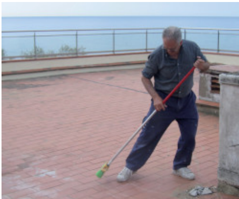
Cleaning a substrate before applying Aquaflex Roof
