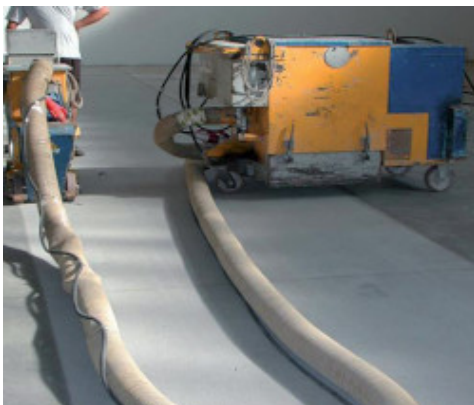
Preparation of the substrate by shot-blasting
