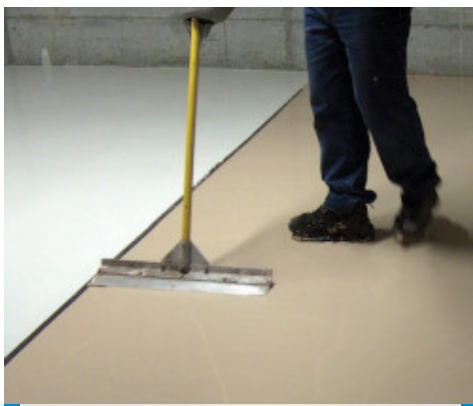
Smoothing Ultratop N immediately after spreading
