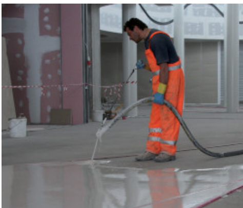
Mechanical application of Ultratop N
