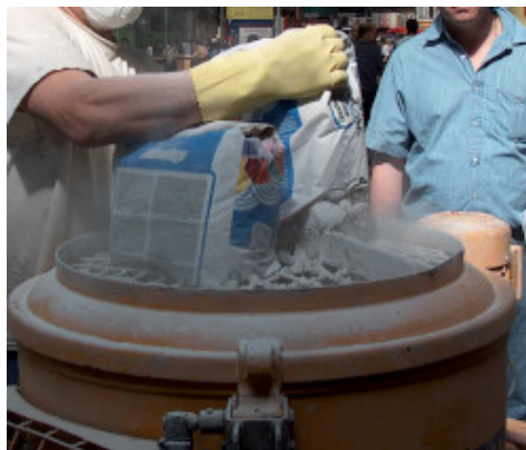
Preparation of Ultratop N in a mixer
