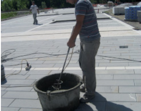
Mix Mapestone PFS 2 Visco only with water using a mixing drill or concrete mixer
