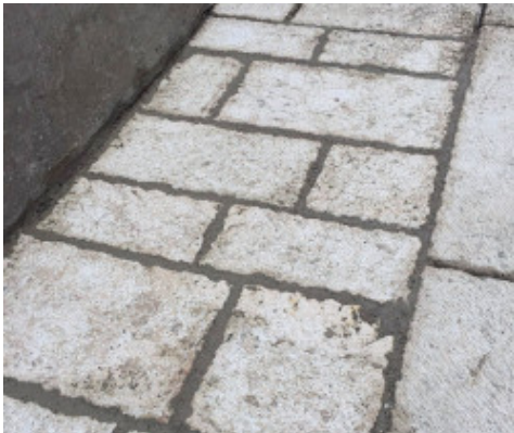
Flagstones grouted with Mapestone PFS 2 Visco
