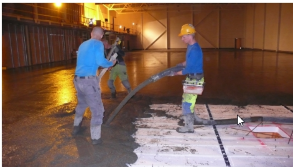
Casting of "Mapecrete System" floor 1300 m 2 jointless
